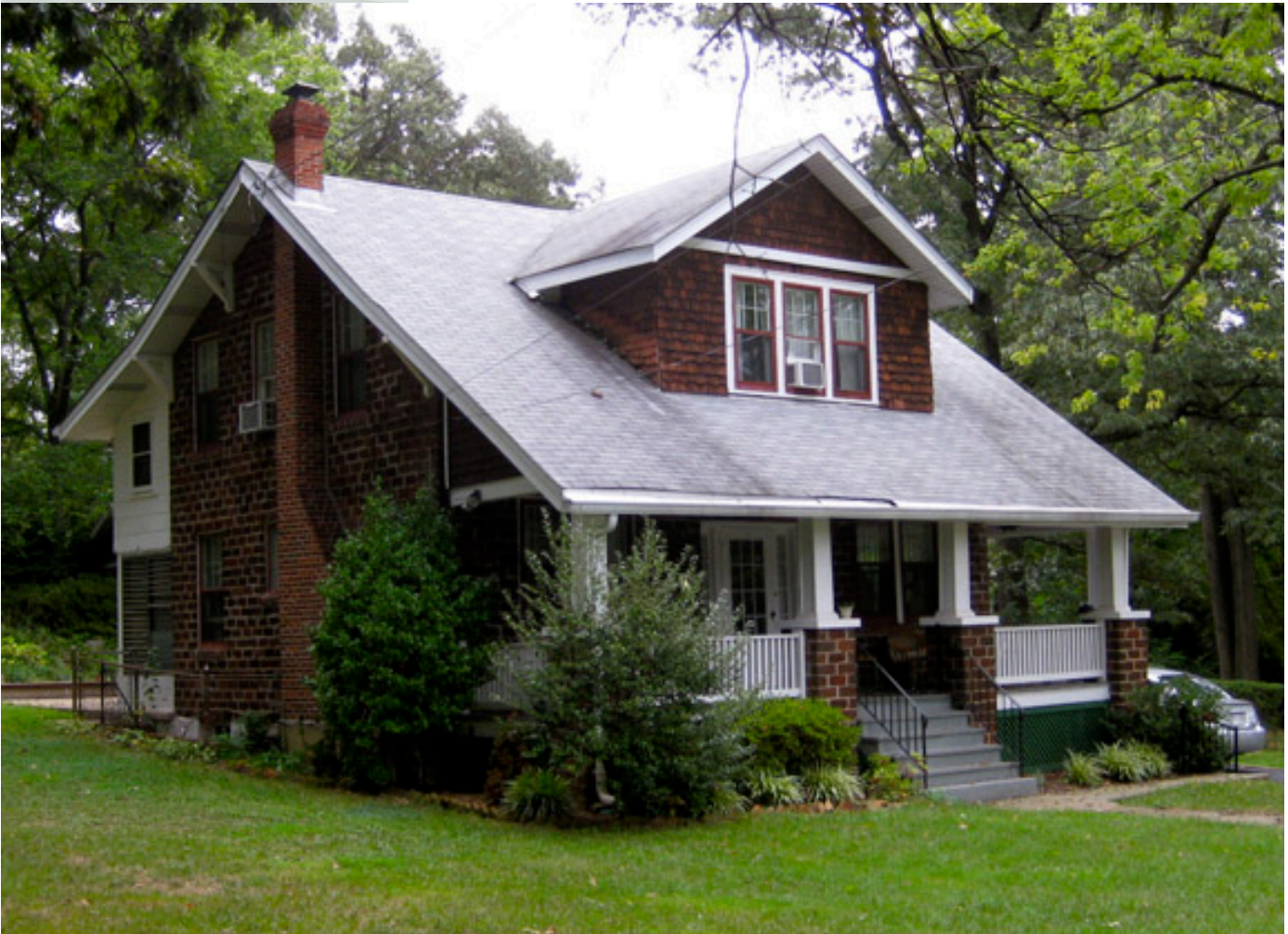
A Craftsman bungalow with a centered gable dormer, brackets under the eaves, and a porch composed of square posts resting on massive brick piers.
