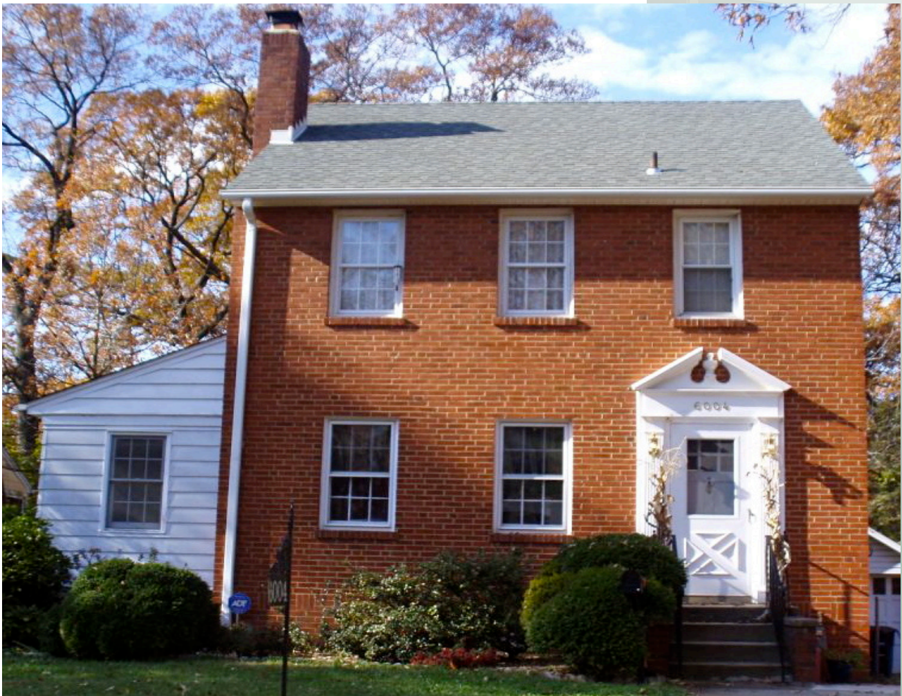
This Colonial Revival displays many of the key features of the style, including a symmetrical façade, six-over-six sash windows, pedimented front entrance and heavy chimney on the gable end.
