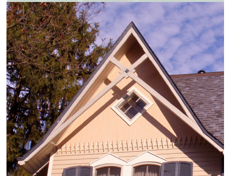
Steeply-pitched gable with embellished truss and flared overhanging eaves.
