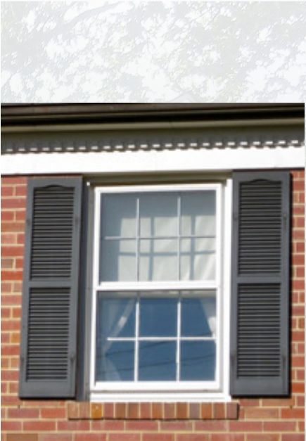
Six-over-six double hung wood windows are one identifying feature of the Colonial Revival style.
