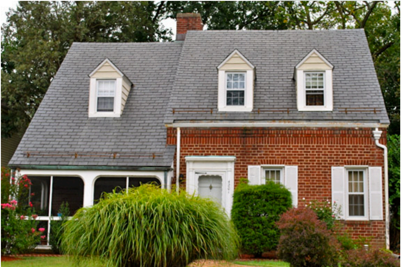
A 1½ story Cape Cod featuring gabled dormers with six-over-six windows, slate roofing, and Flemish bond brick veneer.
