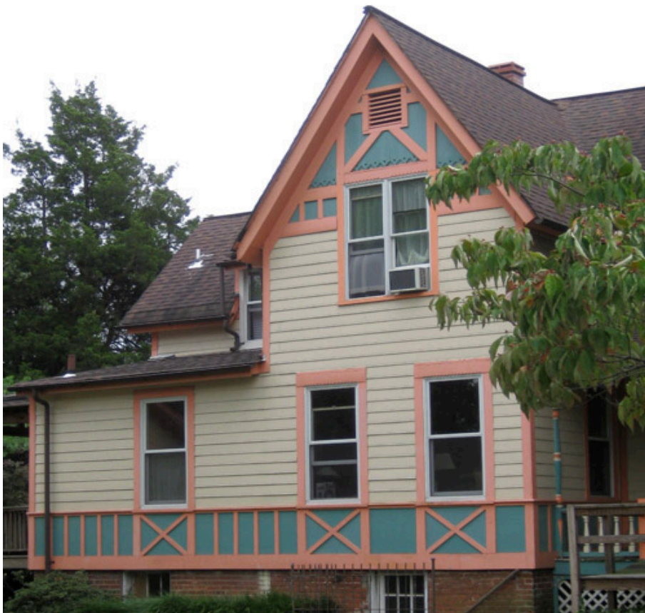
Stick style example showing the juxtaposition of horizontal and vertical siding, combined with the distinctive “X” motif.
