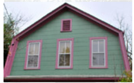
The double pitch of the gambrel roof provides more living space under the gable.
